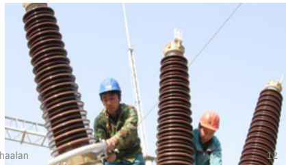
Bushing current transformer installation
